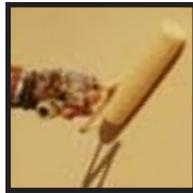
StoGuard™ is an air barrier and a moisture barrier. It prevents condensation related to mass air movement through the wall. In addition, StoGuard cuts off the path for wind-driven rain water to enter the building. As a secondary waterproof barrier bonded to the water sensitive sheathing of the building envelope, StoGuard resists damage and is easily integrated with flashing.
