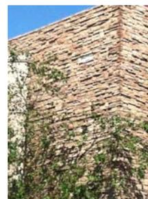
Thin set brick and cultured stone are similar to the stucco and EIFS systems mentioned above. Any water entry can cause freezing and cause the cladding to spall off the
